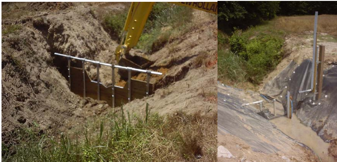
Figure 6. At the central stream site, a plywood board and steel pipe weir was constructed and pushed into the ground with a backhoe. The backhoe can also remove the structure by pulling up on cables attached to the pipes.
